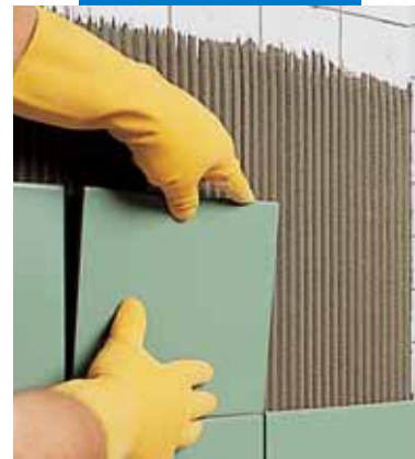
Laying over old tiles
