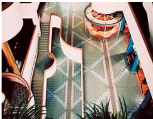
"Porcelain" quarry tiles laid with Kerabond + Isolastic - Civic Center - North York Ontario (Canada)
