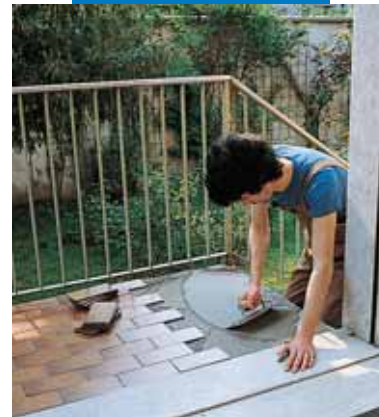
Waterproofing, levelling and laying with Kerabond T + Isolastic
