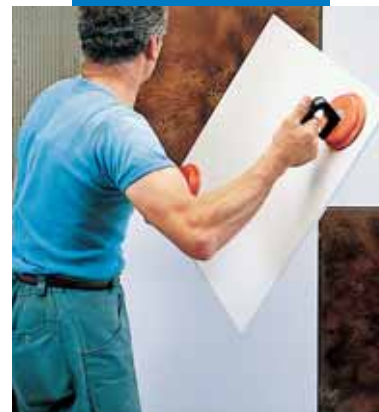
Laying KERAION on a wall
