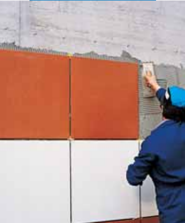
Fixing large size tiles with Kerabond T + Isolastic
