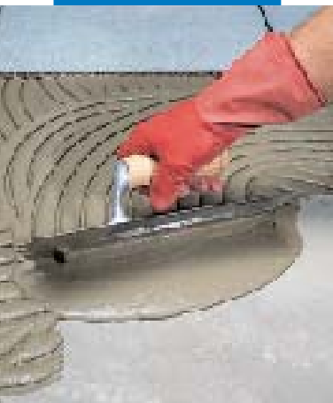
Spreading with semicircular notched trowel
