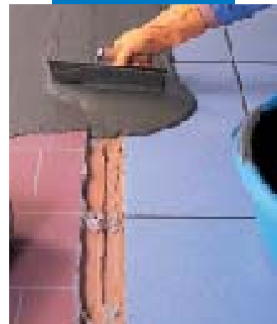
Smoothing existing flooring with Adesilex P4
