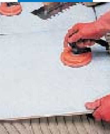
Laying large size tiles
