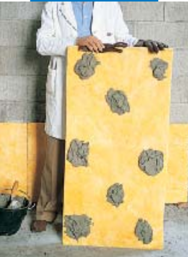
Spot-bonding insulating panels on untreated wall
