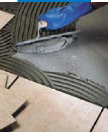
Installation of single-fired tile on floor
