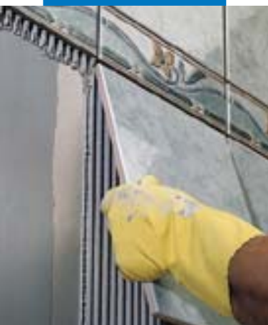
Installation of single-fired tile on wall render
