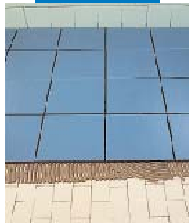
Ceramics onto existing ceramic tiles with Keraflex grey
