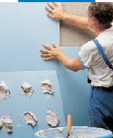
Laying polystyrene foam slabs with Keraflex white
