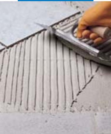
Installation of pre-glossed marble on floors
