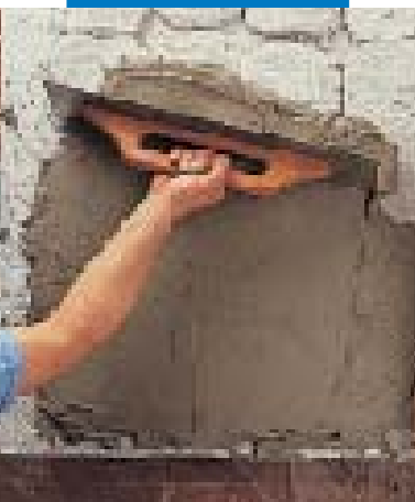
Levelling with a laying-on trowel
