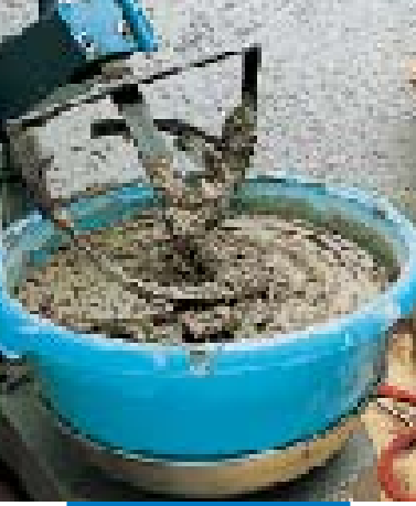
Mixing with a mini cement-mixer
