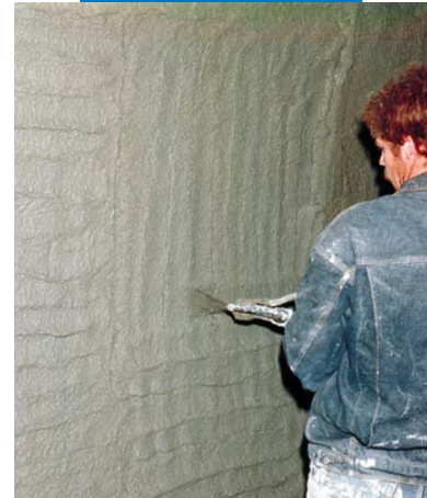
Spray application of Nivoplan
