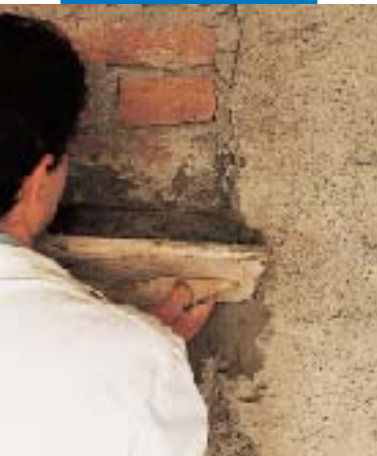
Restoring old brickwork
